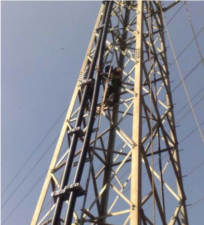
Cable Installation on Ladders
